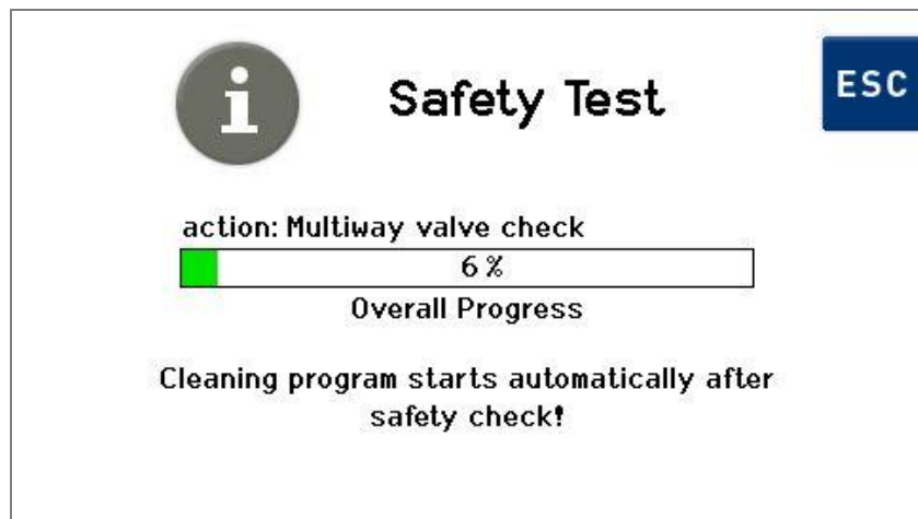
Fig. 10.4.3 Display Safety Test progress
